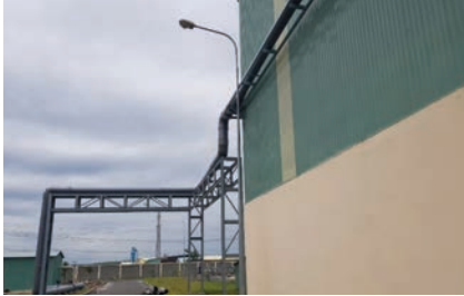
Rainwater Harvesting System (Installed in C&T Vina No.2 Factory)
